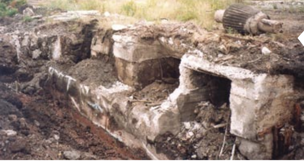
ABANDONED CONCRETE FOUNDATIONS AND SUPPORTS OF POWER PLANT BUILDING AT FORMER CN RAIL CAR SHOPS PROPERTY (JUNE 1997). EXAMPLE OF REMNANTS OF OVER 25 BUILDINGS STILL ON THE SITE IN 1997.
